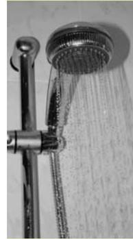
**Use a cloth between the showerhead and the jaws of the wrench to avoid scratching.**
