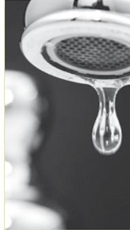
**Water losses** caused by dripping faucets can range from several gallons to hundreds of gallons of water per day. If it is hot water, you're wasting water and the energy required to heat it. Leaky faucets are usually caused by a worn washer or O rings. To fix leaky faucets, you need:
