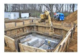
Beginning in November of 2018, the Authority began the complete replacement of the South Temple Sewage Pump Station. The original station was built approximately 1960. As the years passed and development took place, the existing station was at its capacity and needed to be upgraded. Due to a very small footprint, the existing station had no room for expansion and it was decided to build a new station on the same property as the old station. The first photo is the start of construction in
